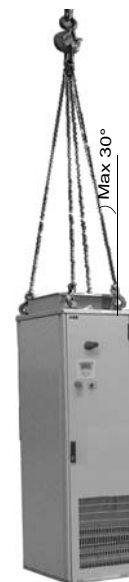
lift the drive by crane
