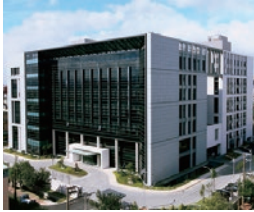
Taoyuan Technology Center (Green Building)
