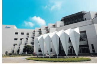
Tainan Plant (Diamond-rated Green Building)
