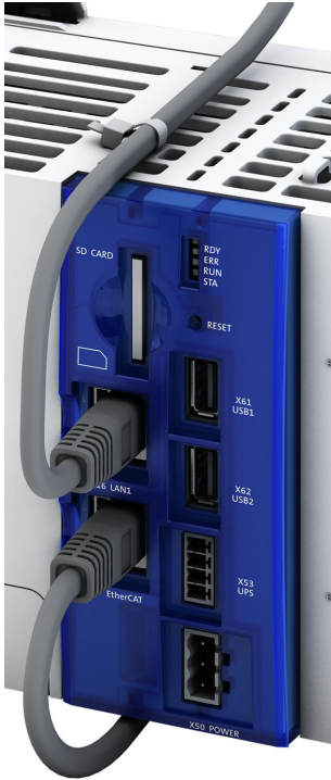
Fig. 1: Installation and fixing of the network cables
