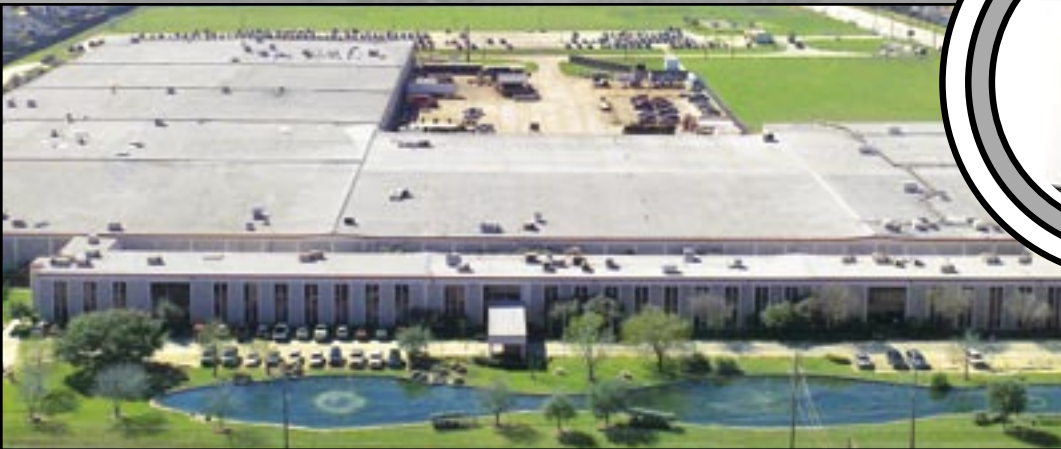
North America Headquarters & Manufacturing Facilities (Houston, TX)
