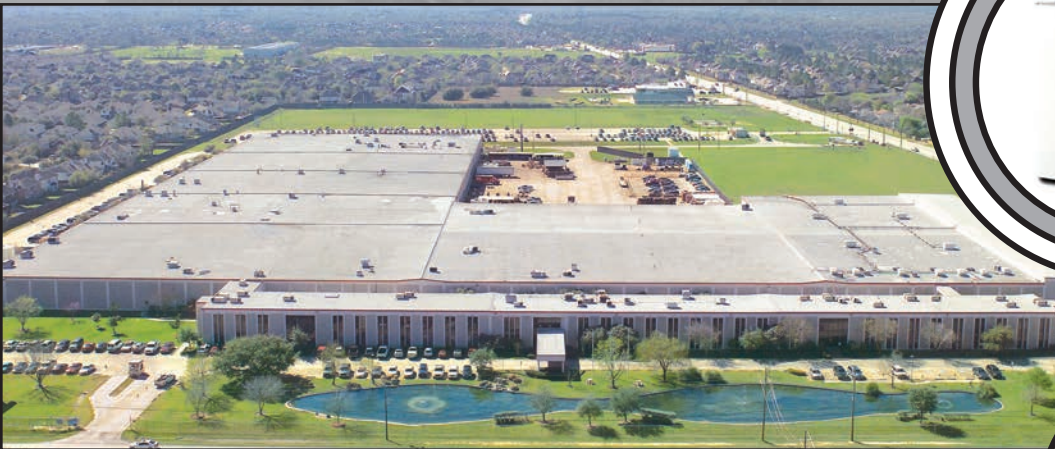
North America Headquarters & Manufacturing Facilities (Houston, TX)
