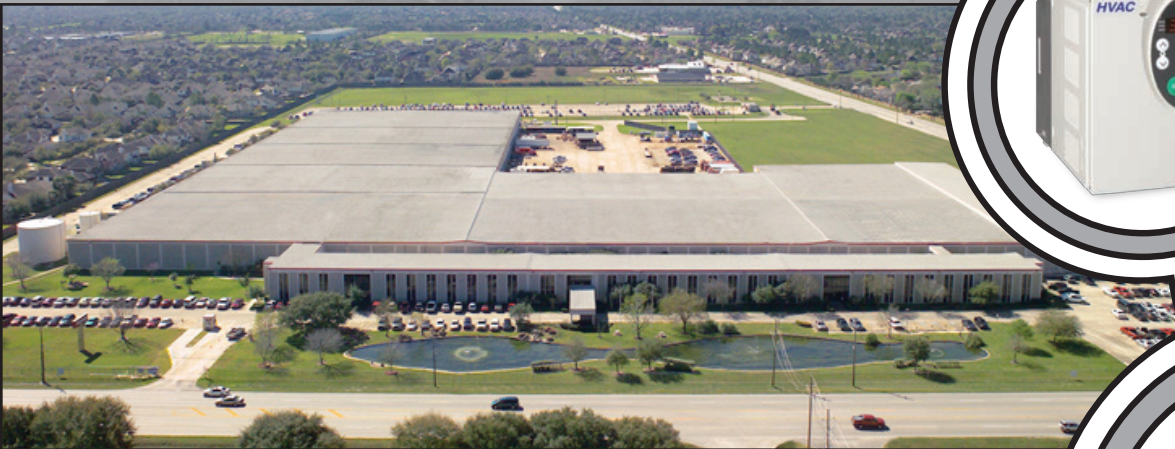
North America Headquarters & Manufacturing Facilities (Houston, TX)
